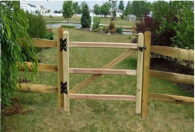
Split Rail Gate Style Example
